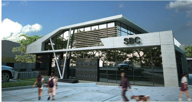
Image 3 Office Building for HVAC equipments in Tbilisi) architect - M. Giorgobiani
