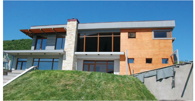
Image 10 Residential House in Mtskheta Realized Architect - M. Giorgobiani
