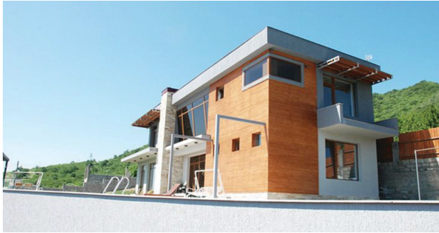
Image 9 Residential House in Mtskheta Realized Architect - M. Giorgobiani
