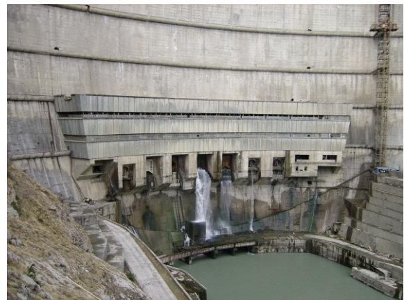
Figure 2. Enguri HPP high-pressure bottom outlet
